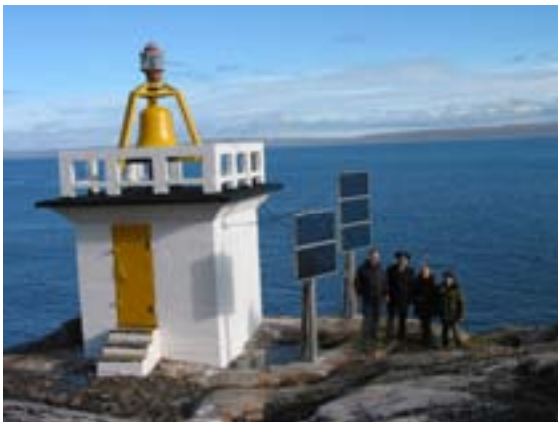
Lighthouse operated by solar cell batteries. Photo: County Governor of Finnmark
