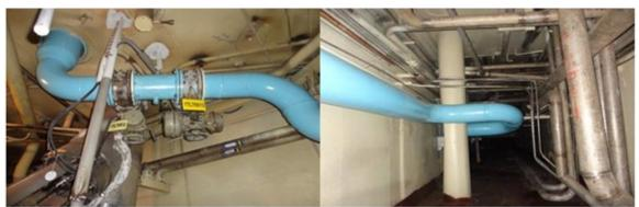
Fig. 3.3 Implementation of the filtered containment venting concept in the event of a severe accident at SUNPP-1
