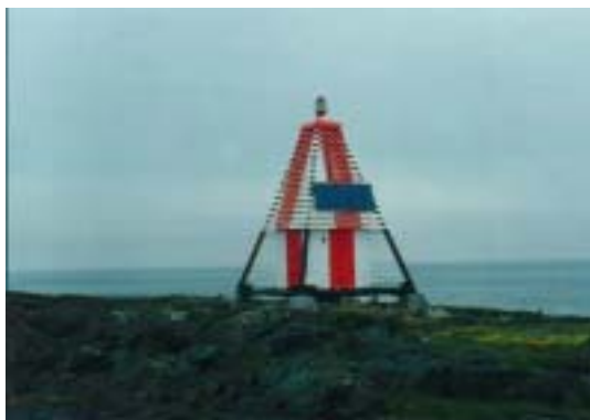
Russian lighthouse at the Kola Peninsula with a solar panel installed. Photo: County Governor's Office, Finnmark
