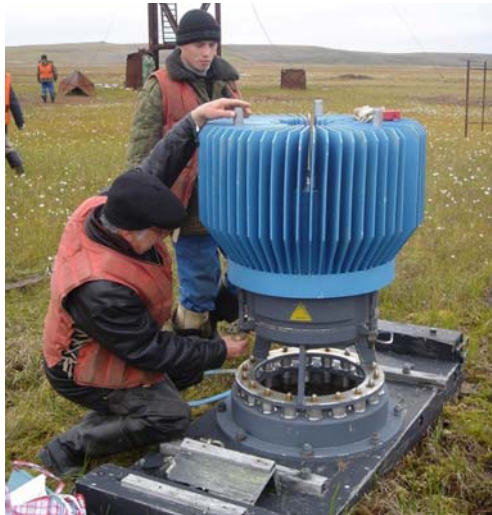
Removal of an RTG from its original placement in Northwest Russia (Photo: County Governor of Finnmark).
