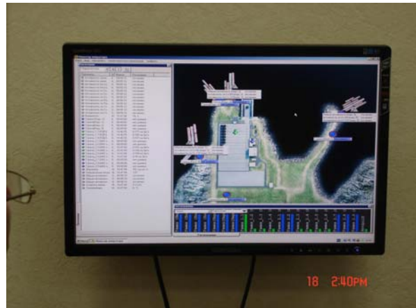
Fig.6 Overview with the monitoring system at Saida
